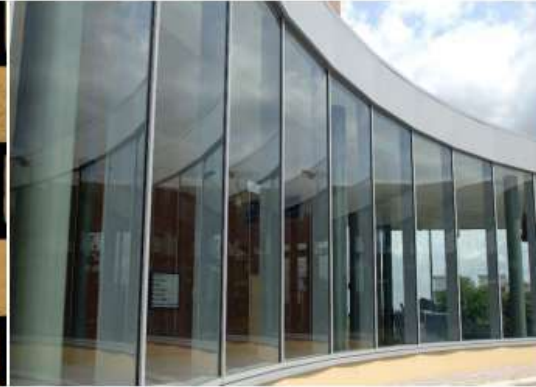
Faceted curtain walling to main entrance
