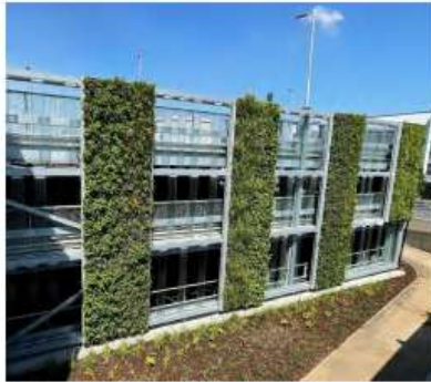
Car park hit-and-miss glass panels and green wall (to match Bedford Avenue carpark) Glass panels: Profilit glass
