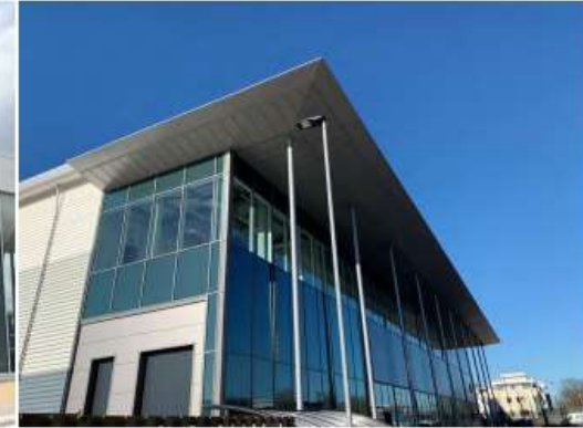
Overhang and curtain walling
