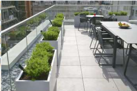
Roof terrace: Structural glass balustrade with stainless steel handrail Porcelain paving tiles
